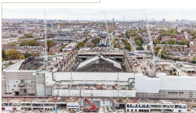
The 1,300 tonne roof of EC1 was lowered in an eleven-hour, precise operation
