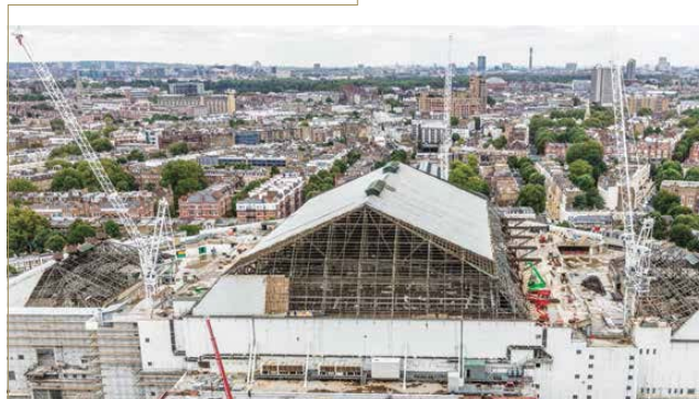
By summer 2015, all internal demolition complete and roof trusses prepared for demolition
