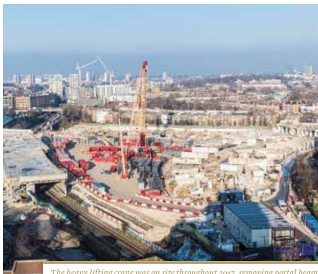
The heavy lifting crane was on site throughout 2017, removing portal beams from site to allow site preparation work to take place
