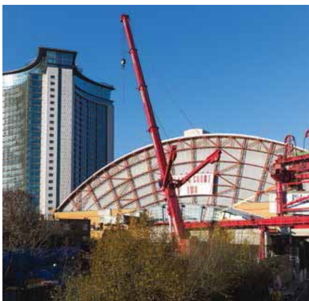
Demolition of Earls Court commences
