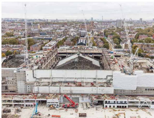
Progress at Earls Court. EC1 roof lowered October 2015
