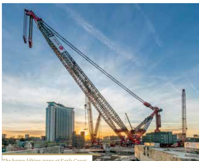
The heavy lifting crane at Earls Court
