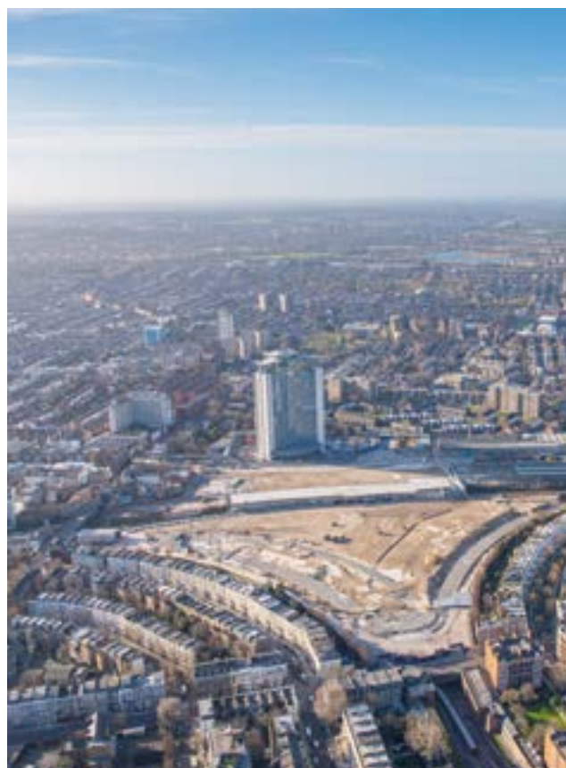
Site progress at Earls Court
